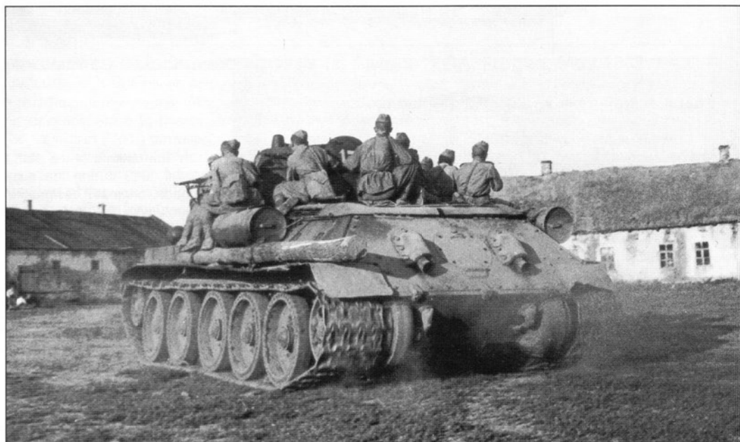
Another view of a group of tank desant on a T-34 Model 1943 near Voroshilovgrad in 1943. The large log on the side of the tank is used to unditch the tank. There were special attachment points on the track for the crew to lash the unditching beam. (N. G. Kolly)
