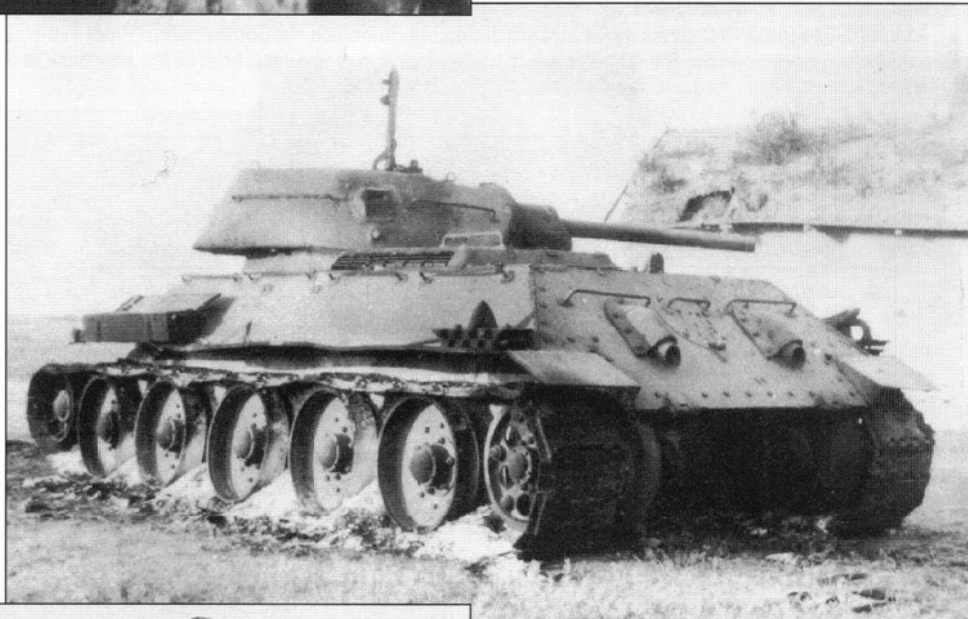
A T-34 Model 1942 knocked out during the fighting on the Southwestern Front in the summer of 1942. This tank has many of the detail features of the vehicles produced at Gorki's Krasnoye Sormovo Plant No. 112, notably its distinctive pattern of infantry hand-holds. This tank has suffered a fire which has completely burned the rubber off the roadwheels. (USNA)
