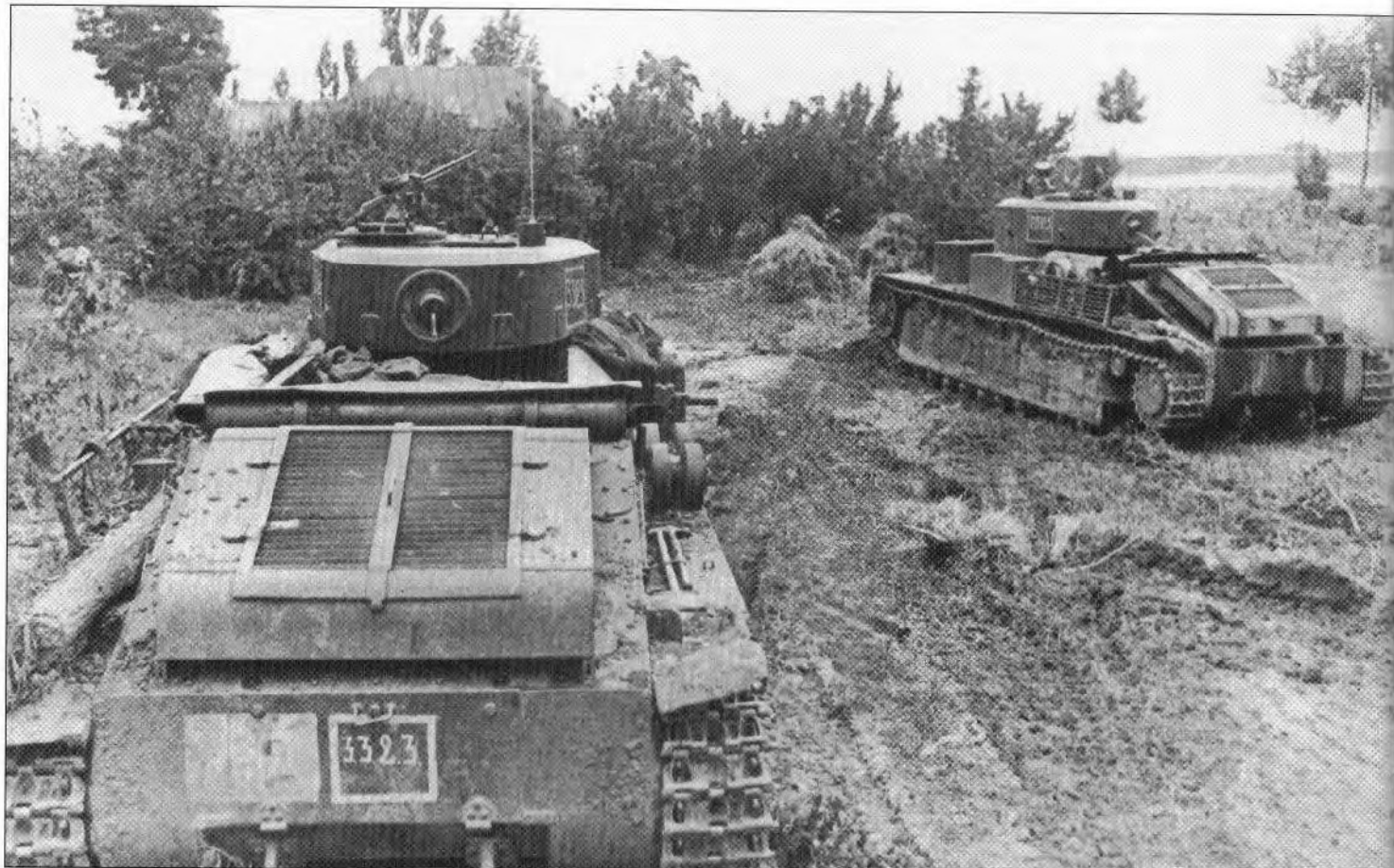
A pair of T-28s go into action in the late summer of 1941. Few T-28s survived the summer 1941 fighting. Both vehicles are fitted with the standard P-40 anti-aircraft machine gun mounting on the roof, and the nearest vehicle has the later style whip radio antenna instead of the more common "clothes-line" antenna. These T-28s have an unusual tactical marking consisting of a four-digit number in a rectangle, and the nearest tank also has a large white rectangle at the rear.
