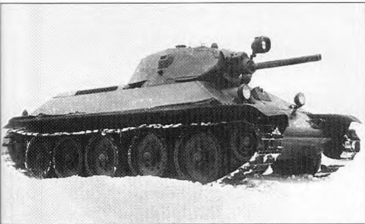
One of the prototypes of the T-34 Model 1940 is seen here during trials at the NIIBT (Scientific Research Institute for Armor Technology) at Kubinka in the Moscow region during 1940. The prototype differs from the series production vehicles in many details including the absence of much of the hull tool stowage, the armor strips around the driver's hatch and other features. Although the series production tanks retained the mounting lug for the tank gun search light, it was seldom, if ever, fit on production vehicles. (NIIBT Archive, Kubinka)
