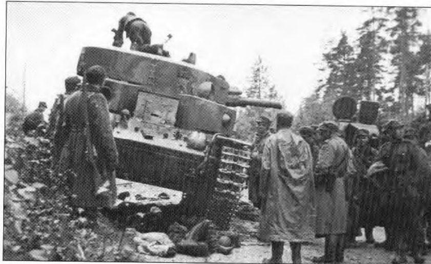
Finnish troops inspect a T-28 Model 1938 knocked out near Prassa on the Karelian isthmus in September 1941. This is one of the late production vehicles fitted with the improved L-10 76.2mm tank gun which gave better anti-armor performance.
