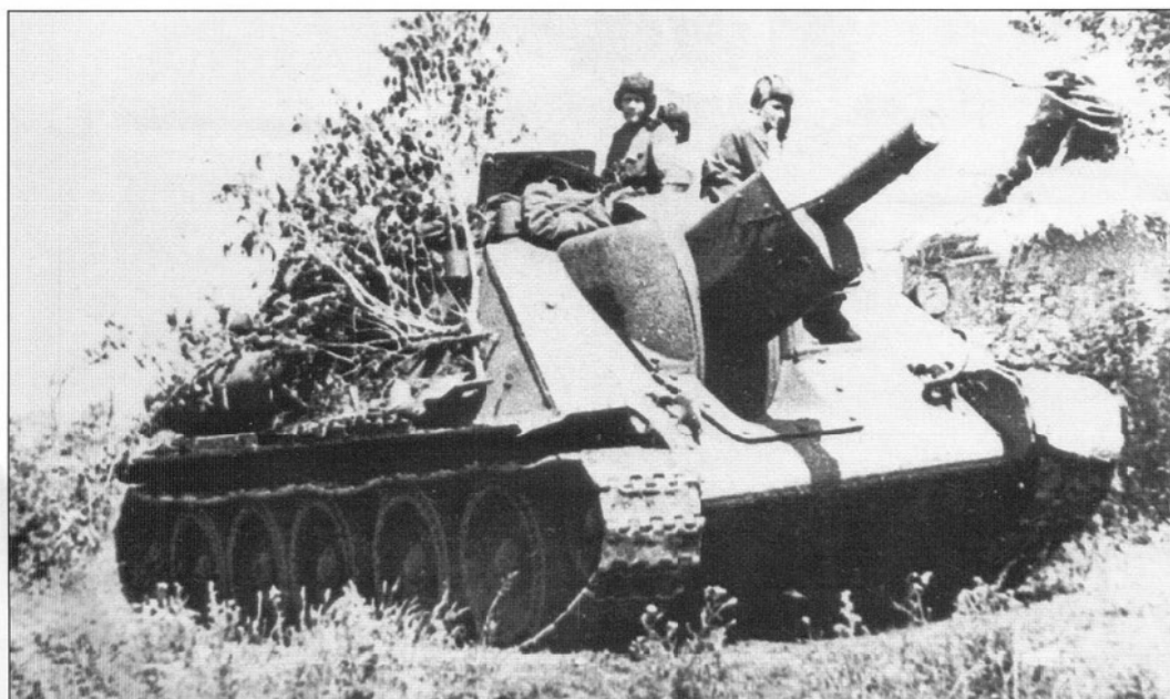
The success of the German StuG III Sturmgeschutz prompted the Soviets to develop a similar vehicle, the SU-122. This was armed with a 122mm M-30 howitzer in a fixed casemate. These vehicles were intended to provide direct fire support during infantry operations.
