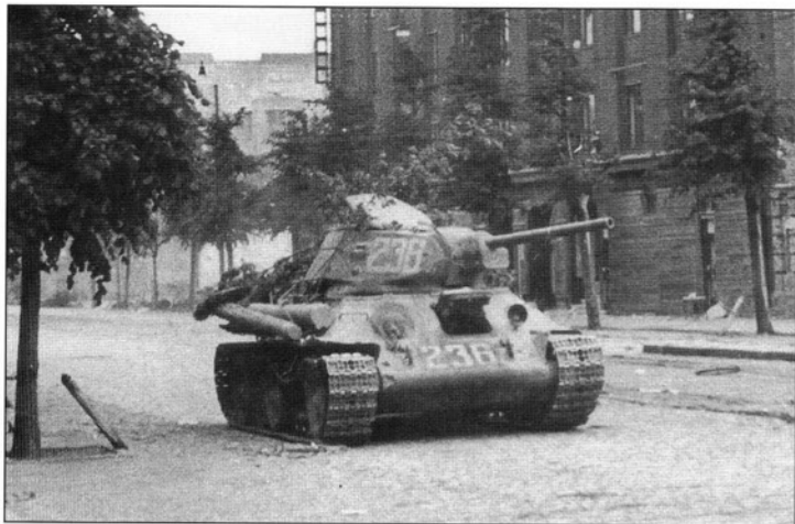
Another tank from the same unit is seen on the streets of Vyborg on 20 June 1944. This is a war-weary old T-34 Model 1942- note that it is missing its number 2 and 4 road-wheels. All the tanks of this unit carried the three digit tactical number on the glacis plate as well as on the turret sides. (Suchatov)
