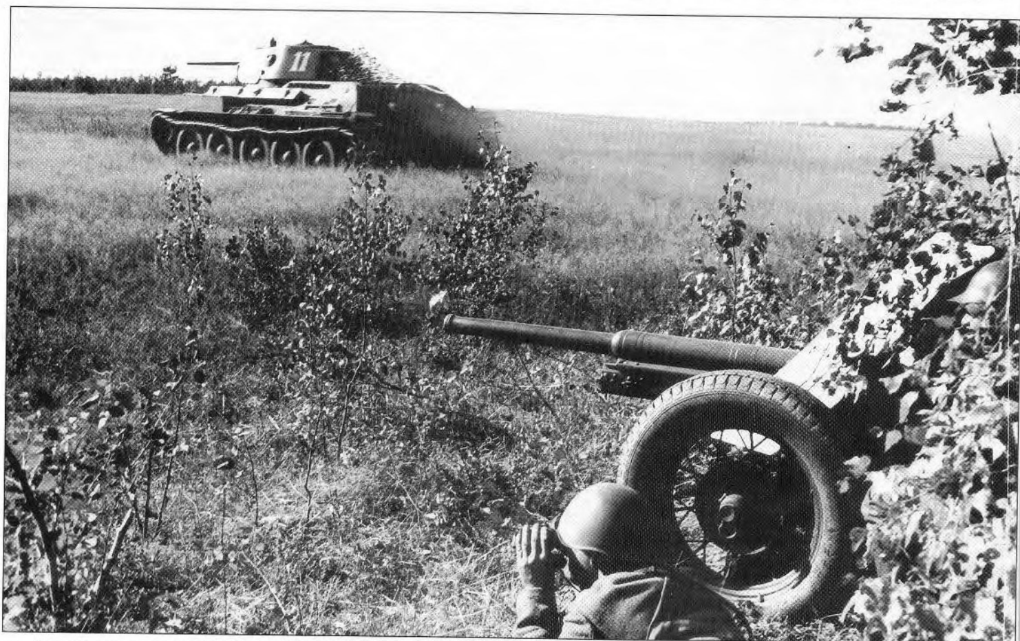
A rare view of a T-34 Model 1941 moving into combat on the Western Front in the summer of 1941. In the foreground is a 45mm Model 1932 anti-tank gun, the standard Red Army anti-tank gun of this period. The T-34 Model 1941 differed from its predecessor the Model 1940 in the gun; the short L-11 76.2mm gun was replaced by the improved F-34 76.2mm gun which gave it better anti-tank performance. (Petrusov)
