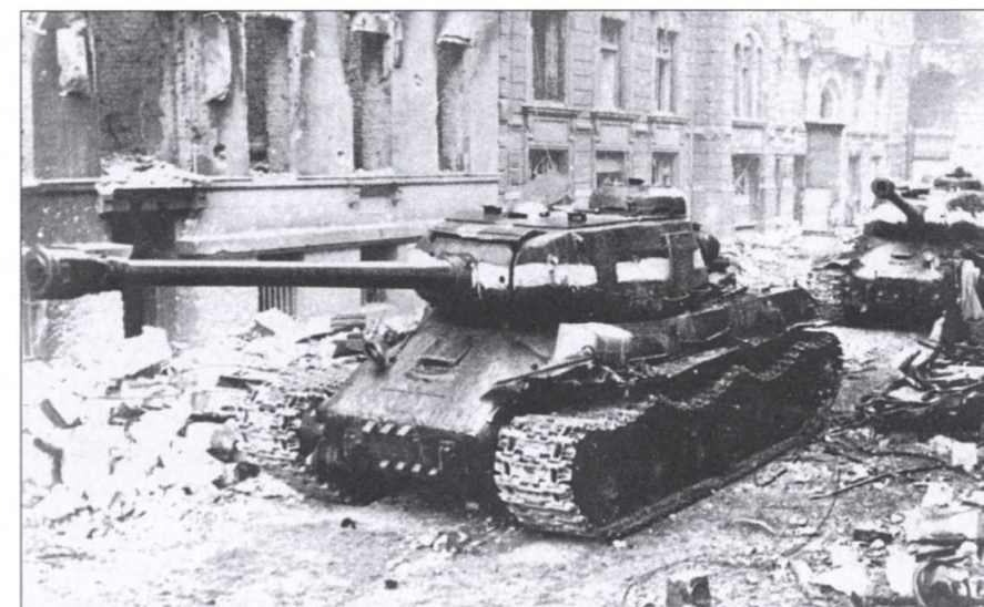
Another of the outcomes of the Kursk fighting was the decision to abandon the KV heavy tanks for a completely redesigned type, the IS-2 Stalin heavy tank. The IS-2 was an evolutionary development of the KV, using a related chassis and engine, but with a radically improved armour layout and new 122mm gun. Unlike the German Tiger I which was optimized for tank-versus-tank fighting, the IS-2 was intended to assist in offensive operations, in both the breakthrough and exploitation phases.
