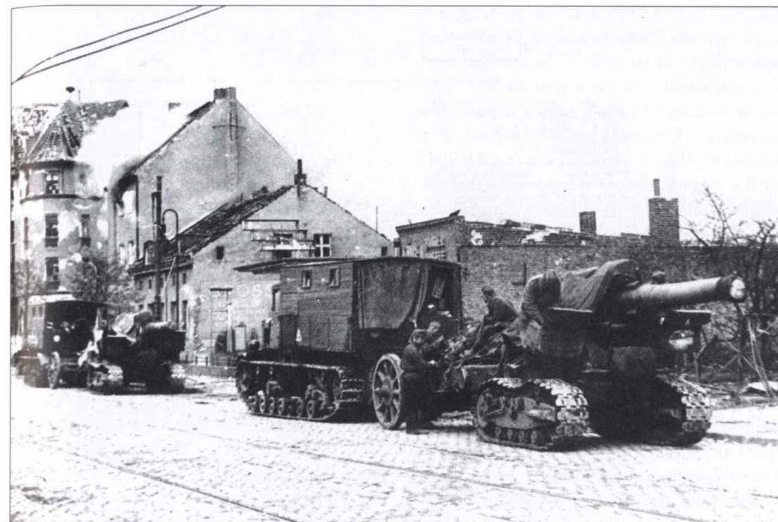
The heaviest artillery was placed in special RVGK Supreme Command Reserve formations which allowed the Red Army to concentrate its firepower and missions. Here, a pair of 203mm B-4 Model 1931 howitzers are towed by Voroshilovets artillery tractors. The BR-2 used an unusual tracked undercarriage to better distribute its heavy weight – the undercarriage was not powered.
