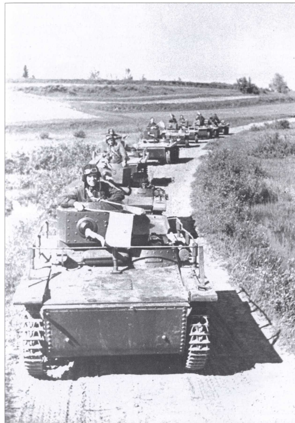
A column of T-37 amphibious tanks on the move. These small, machine gun-armed vehicles were designed for scouting. Few survived the devastating battles of the summer of 1941 and the Red Army gave up on the luxury of amphibious scout tanks until after the war.
