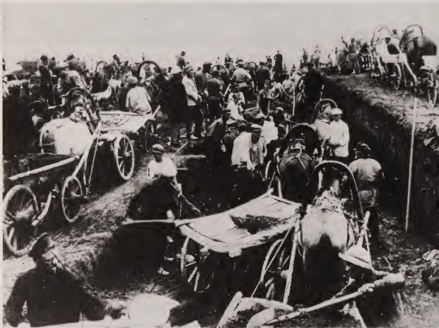
Constructing the Chelyabinsk Tractor Works during the early five-year plans. Construction in the early period often relied on primitive techniques and mass labour (SCR)
