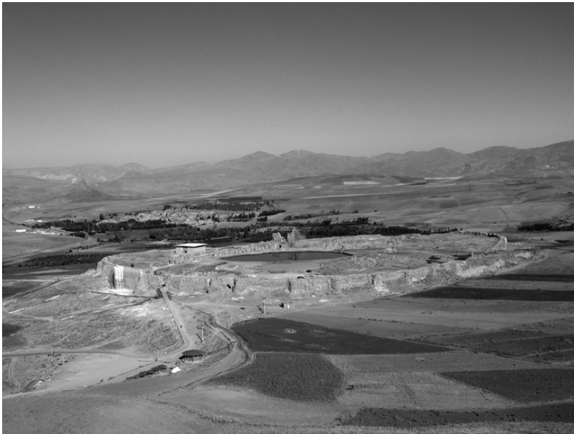
Figure 18.1 Takht-i Sulaymān, general view. Photograph: Yousef Moradi
