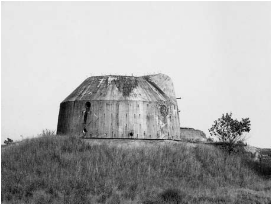
Experimental mobile bunker: The upper mass pivots on its base and shows alternately its open face during firing and its blind side for protection after firing.
