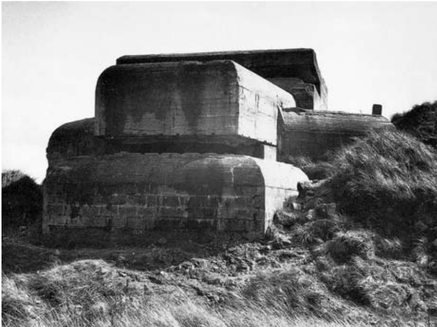
Two types of facades: The upper slab protects the telemeter, which controls the firing in the battery; the lower slab protects the command.
