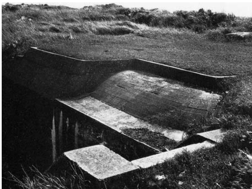
top: Simple concrete trench for six to eight soldiers bottom: Architectural details for a banquette
