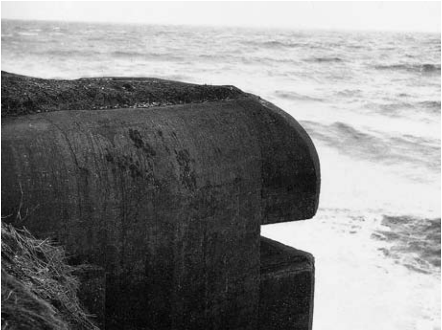
top: Bunker with two embrasures: This type of fortification is rare on account of multiple concealment problems. bottom: Lookout post
