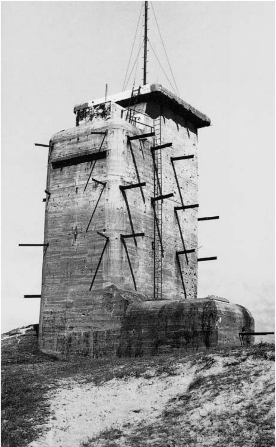
Firing direction tower in Brittany: The steel beams sticking out of this bunker are there to provoke premature explosion of projectiles before they hit the fortification.
