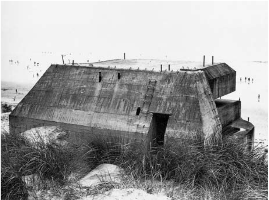
top: Command post in the south of Brittany bottom: The rear solid mass of a firing control post
