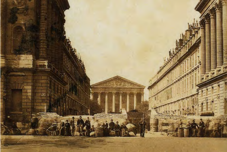
A Barricade on the new Haussmannian Avenue de la Madeleine during the 1871 Paris' Commune
