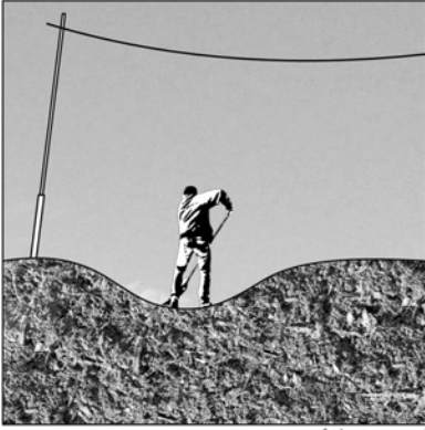
excavation of the ground
