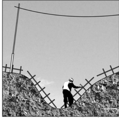
reinforcement bars placement
