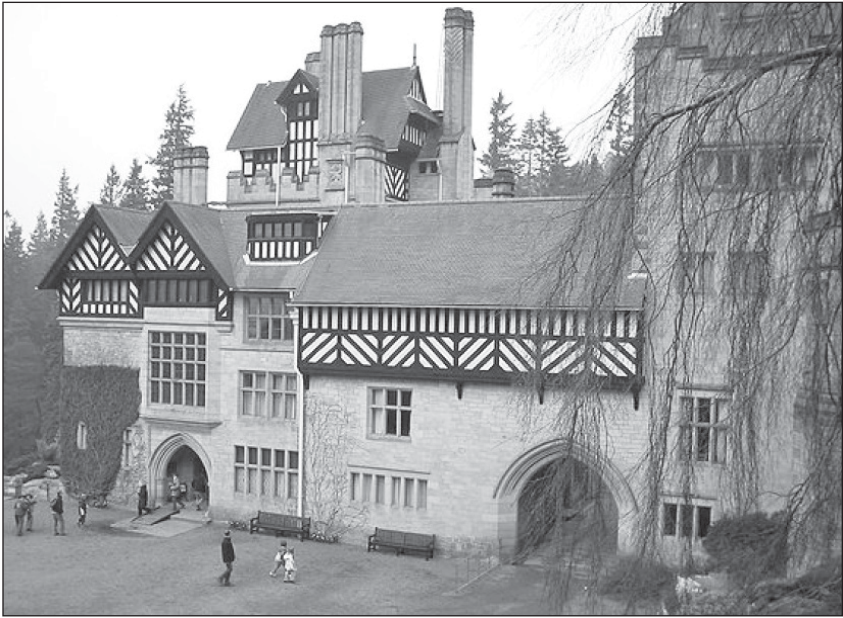
Figure 5.33. Cragside House, constructed for the Newcastle armaments manufacturer William George Armstrong, later Lord Armstrong. Photo: Dave Sumpner, English Wikipedia.
