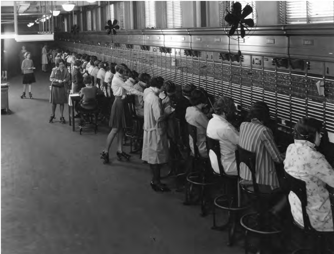
Figure 1.5 The Chicago Long-Distance (Toll) Office in 1929. (Source: Courtesy of AT&T Archives and History Center.)
