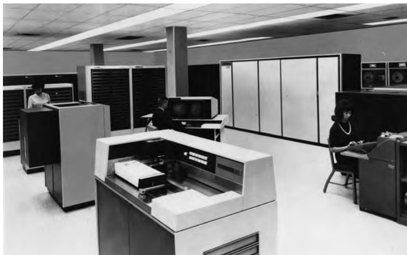
Figure 5.7 A Control Data Corporation 6400 with a 405 card reader in foreground, 1965. (Source: Image courtesy of the Charles Babbage Institute Archives, University of Minnesota Libraries, Minneapolis.)
